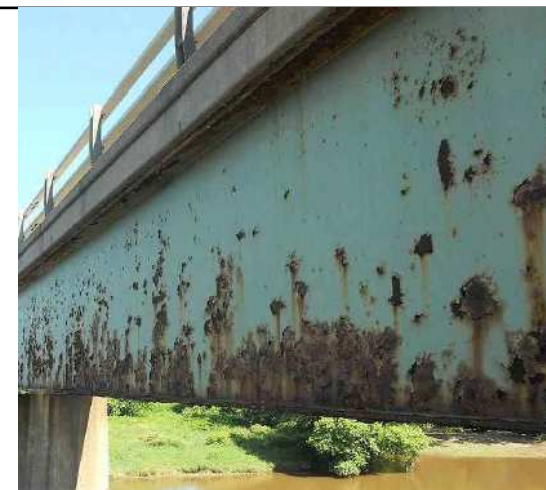
Fonte: BRIDGE INSPECTION MANUAL – NY'S DOT
