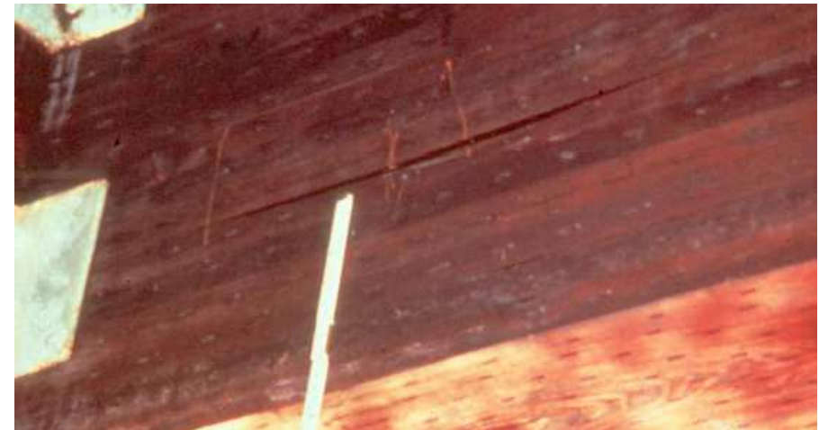
Fonte: BRIDGE INSPECTION MANUAL – NY'S DOT
